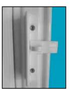
2. Then slam the door. Once closed, place the locking latch as indicated in the picture until it stops at the closure.
